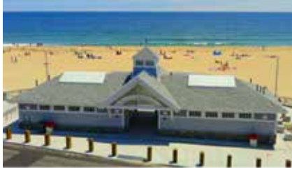
Marine Memorial & North Bathhouse
